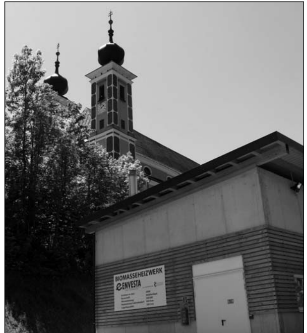
Biomass operations in Austria are integrated into the rural landscape. Here an energy facility is neatly run next door to a historic 12th century cathedral. Clean-burning stoves greatly reduce airborne pollutants.
